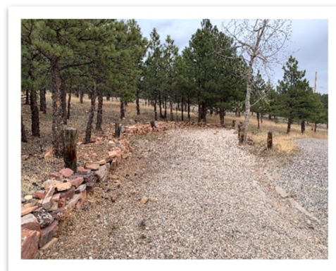
Stone Wall & Bollard Repair
